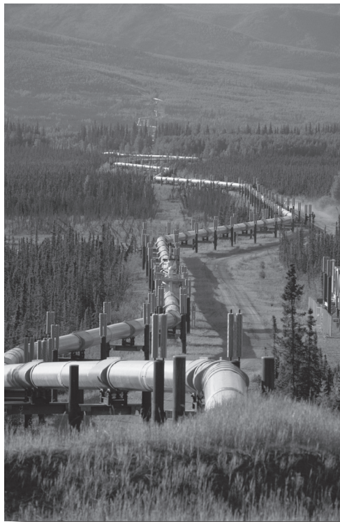
Trans Alaska Pipeline through interior Alaska © 2000 AlaskaStock.com
